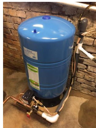
Installation of the 2022 Council. The new pressure tank that brings water from our well.
