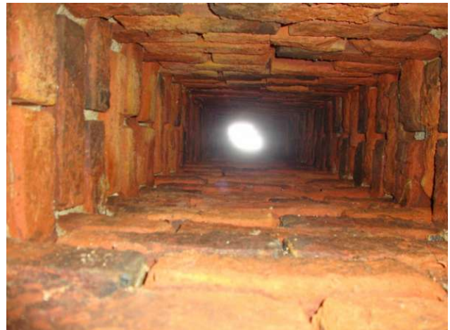
View looking up the Salem chimney after cleaning.
